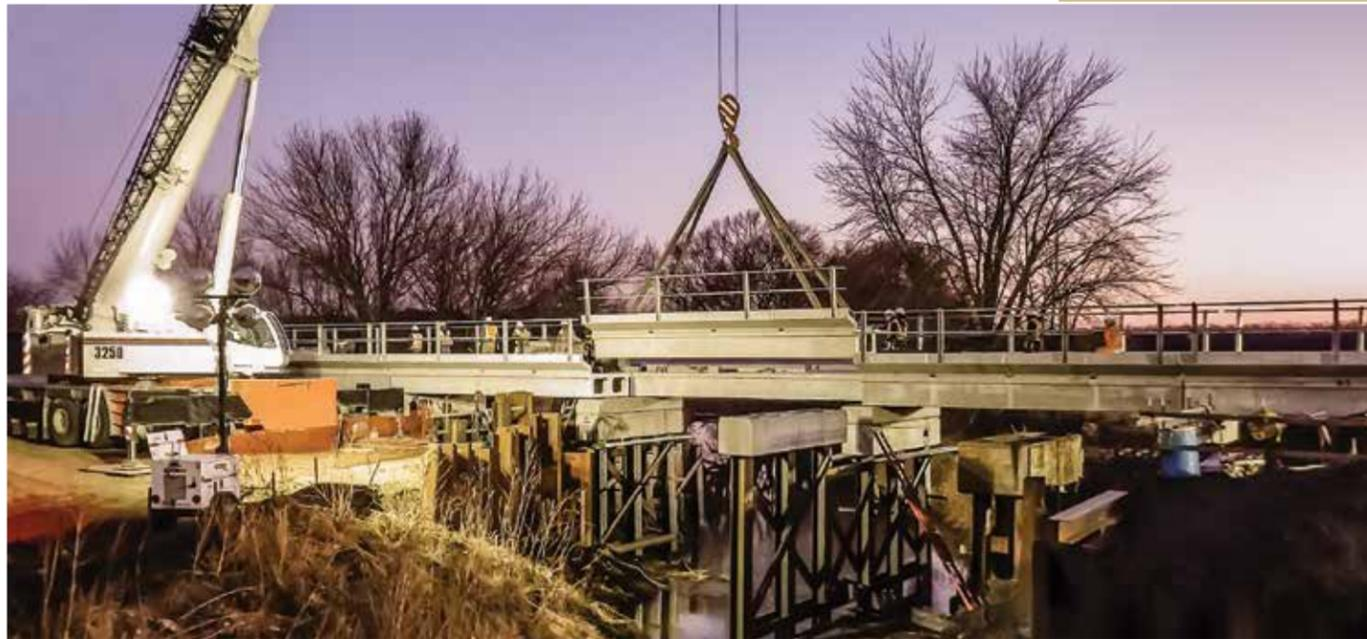
This double track project involved the removal and replacement of a 200-foot bridge within an 18-hour shutdown window.
