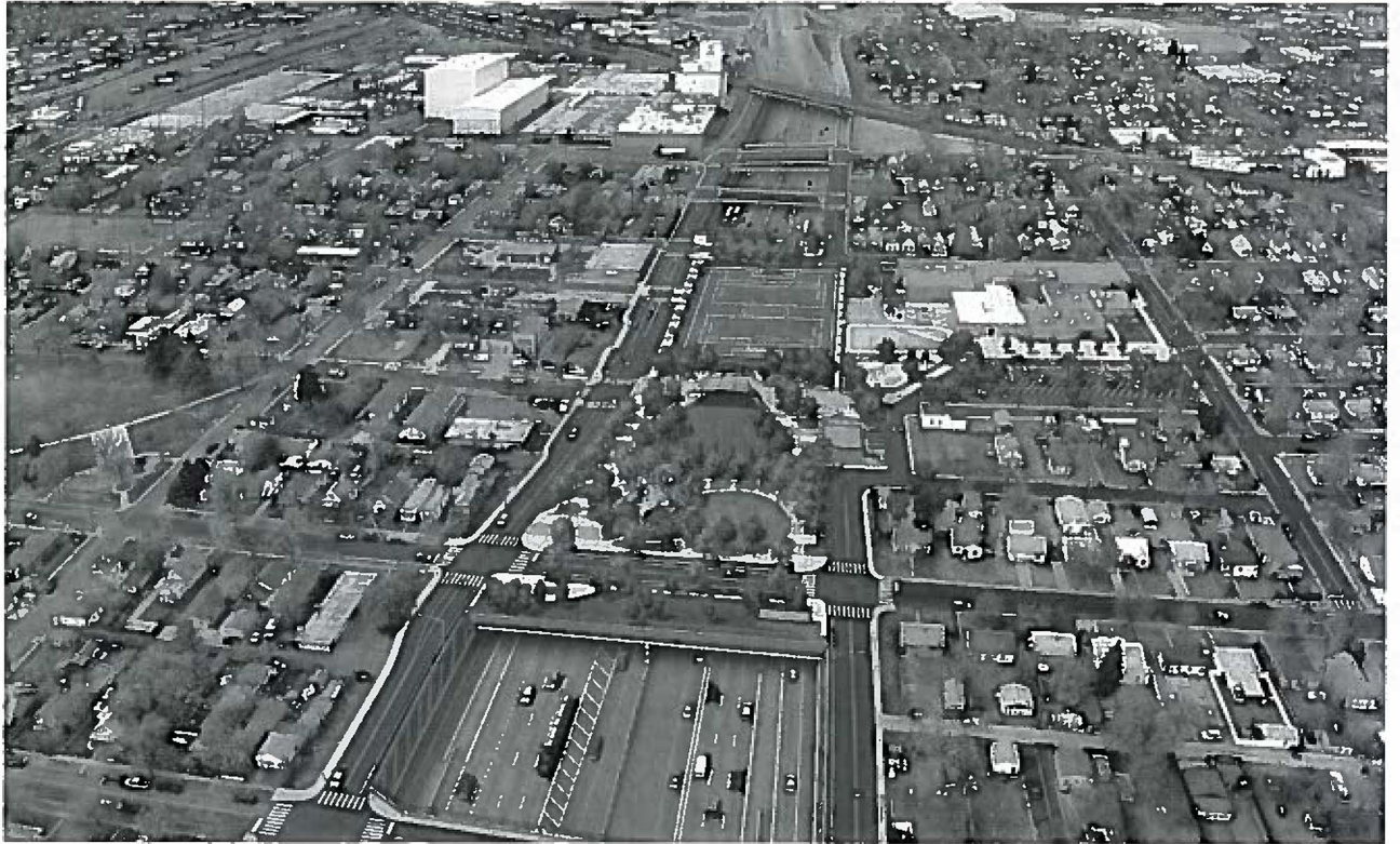
A key element of the Central 70 project is the construction of a four-acre cap, or cover, over the interstate between Clayton and Columbine streets near Swansea Elementary School. Photo courtesy of CDOT
