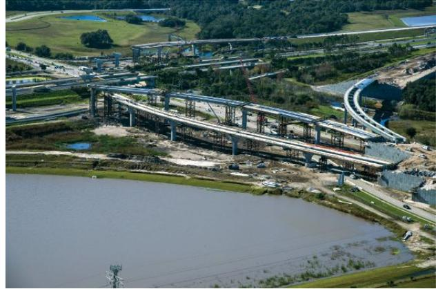
The S.R. 417-South Access Road-Boggy Creek Road interchange project in Orlando, Fla., included the first use of precast concrete U-girders in the state. The four-level interchange and widening of S.R. 417 has improved local traffic conditions and created direct access to Orlando International Airport.
