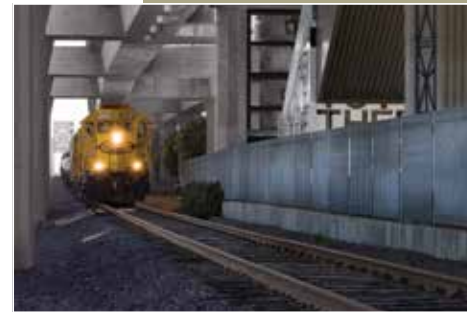
Douglas Street Gap Closure Railroad Grade Separation – Los Angeles, California
