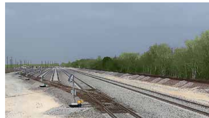
Jefferson Davis Support Yard Project – Lacassine, Louisiana
